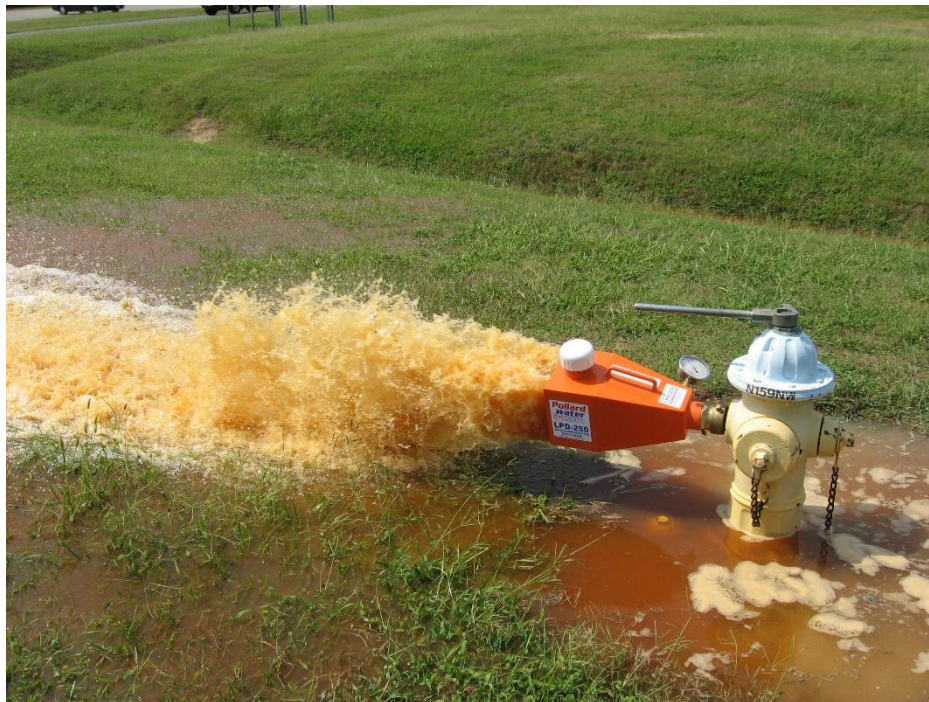
Figure 1-1 Example of Debris Being Flushed Using UDF
