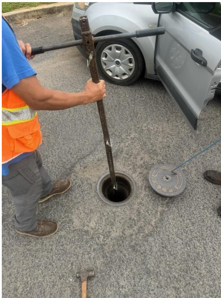
Figure 3-5 Valve Exercise Example
